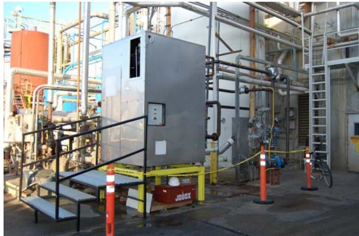
This demonstration unit is designed to supply 75-tons of chilling at the full temperature spread necessary for poultry processing. With a lesser temperature spread, made possible when only “pre-chilling” and “pre-heating” are required, and the existing equipment completes the chilling and heating, then the design capacity increases to 100-tons chilling. Initial operation has been at about 82% of design capacity, and
